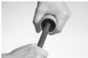
DEBURRING THE TUBE
