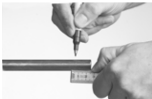
MARKING THE INSERTION DEPTH
