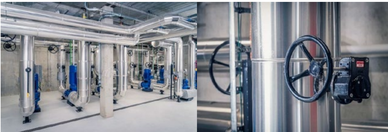
BROEN Ballomax® ball valves controlling the flow of district heating water
