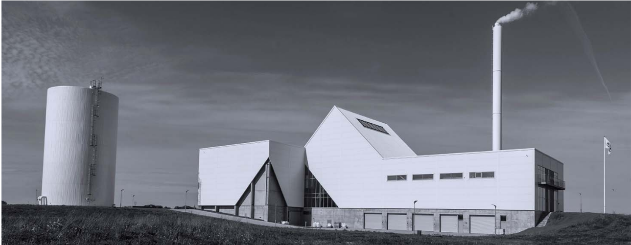
Aabybro district heating plant (Denmark).
