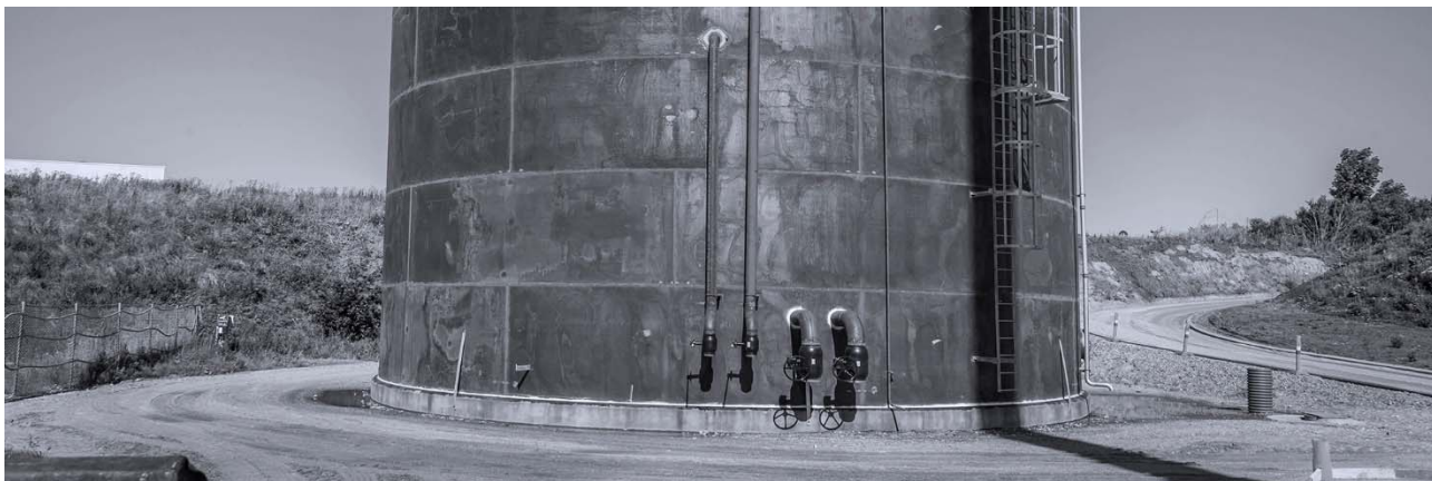
Hobro District Heating Station – a new district heating station with BROEN Ballomax® valves.
