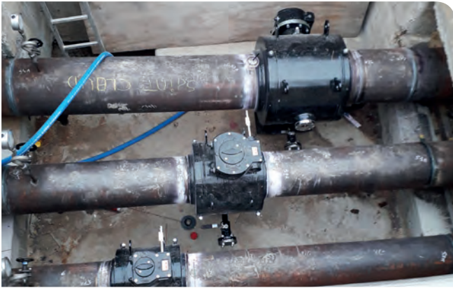
Installation of BROEN Ballomax® Trunnion ball valves in a hot underground water loop on the Paris IDF heat network, EN488:2015 EHP003.
