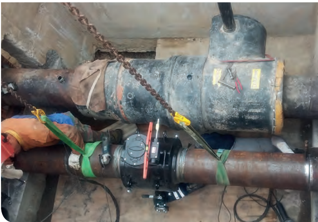
Valve chamber around BROEN Ballomax® Trunnion ball valves for underground installation.
