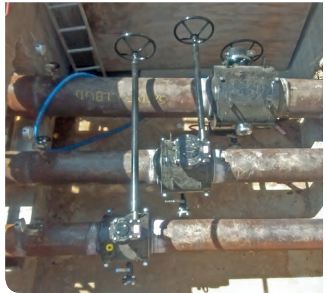
Flexible solution of operation of 3 underground BROEN Ballomax® Trunnion ball valves in a tight space.
